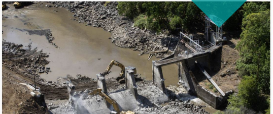
Copco 2 Deconstruction Begins on Klamath River
